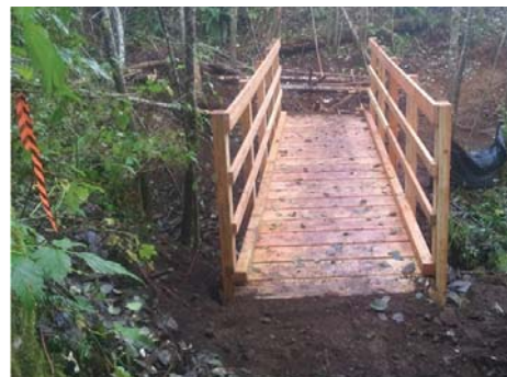
Spaur Creek Bridge © Image by Tom Niemela
